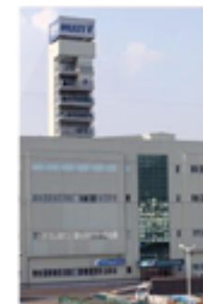
Long Piping and Elevation Testing
